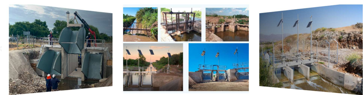
Figura 9: compuertas Flume Gate
