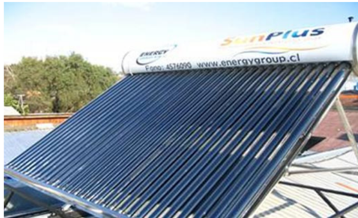
Colector solar tubular
